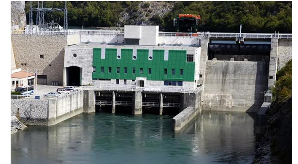
Hydro Power Plant in Croatia (HEP)
