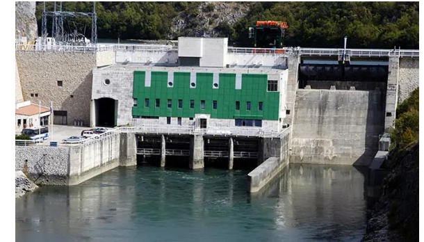
Hydro Power Plant in Croatia (HEP)
