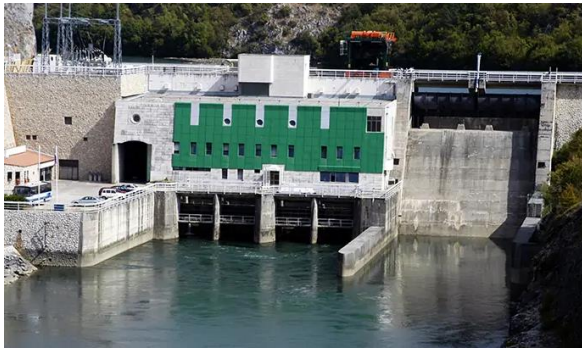
Hydro Power Plant in Croatia (HEP)
